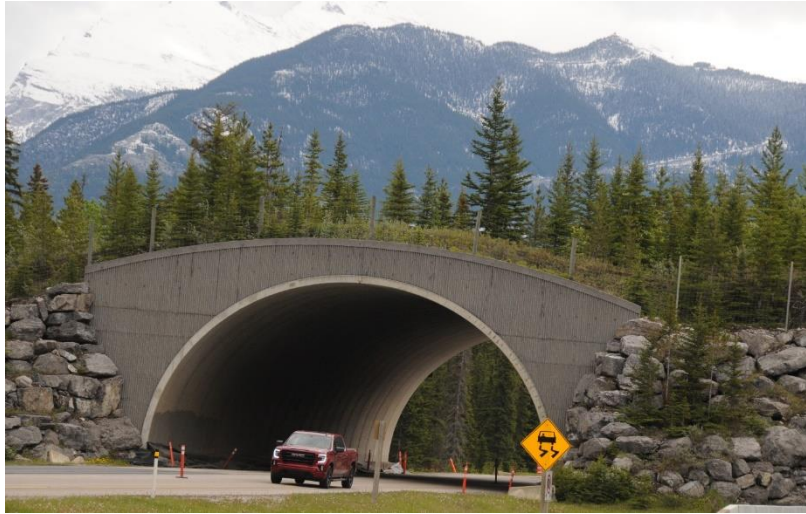
Figure 4. A wildlife crossing structure over the Trans-Canada Highway, Banff National Park, Alberta, Canada (Photo: G. Proulx©).
